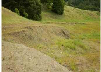
Photo 10: Image of SLIDE showing part of the headscarp and displaced wattles.
